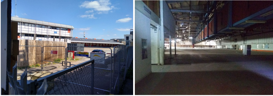
Figure 19 - External and internal views of the existing former sorting office (09/05/2019)
