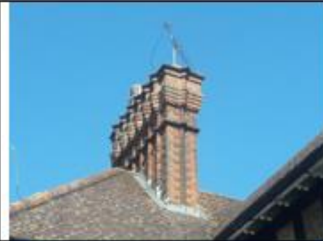
Keepers building, Chimney detail. Photo: Cllr Williams
