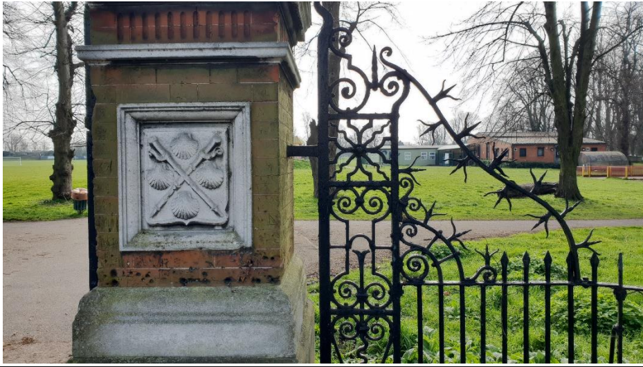
Fig. 7: Entrance gate to park from London Road
