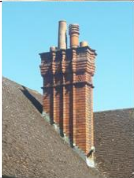
Pavilion building, Chimney detail. Photo: Cllr Williams
